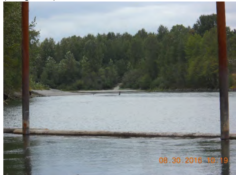
Photo 8 – Looking upstream from end of boarding floats
