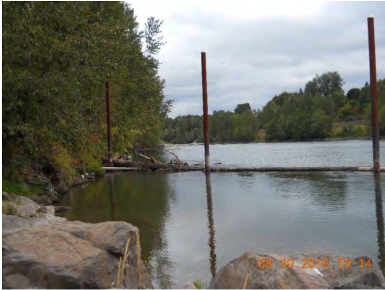
Photo 5 – Pile and log debris deflector
