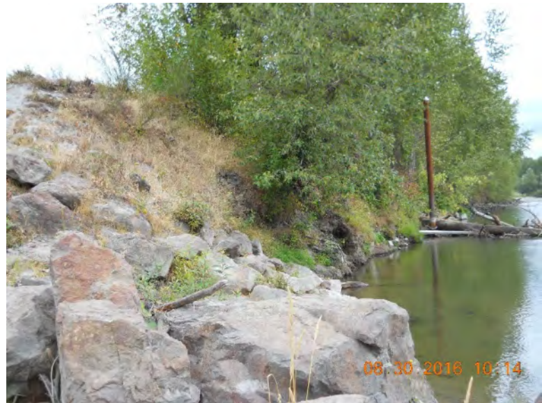
Photo 4 – Looking upstream along left bank
