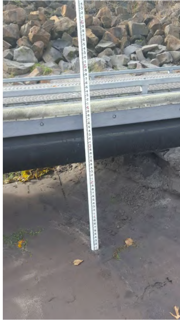
Photo 14 – Sediment deposits from December 9, 2015 high water
