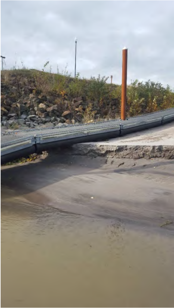
Photo 13 – Sediment deposits from December 9, 2015 high water
