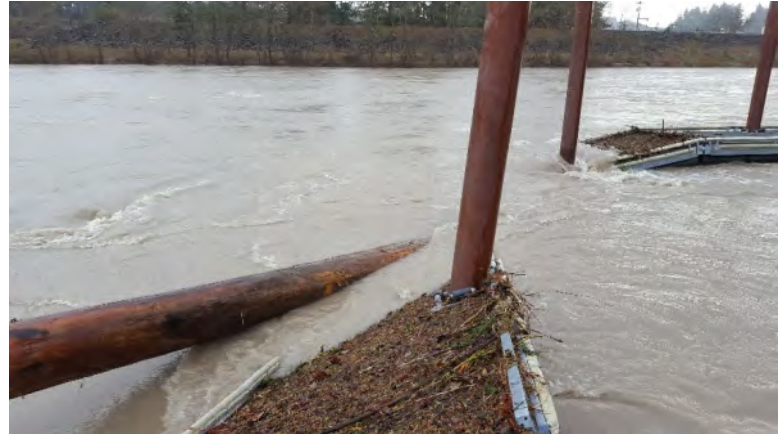
Photo 16 – Debris on floats during December 9, 2015 high water
