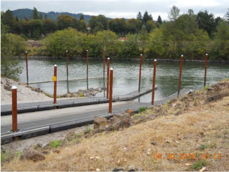
Photo 1 – View of boat ramp from parking area
