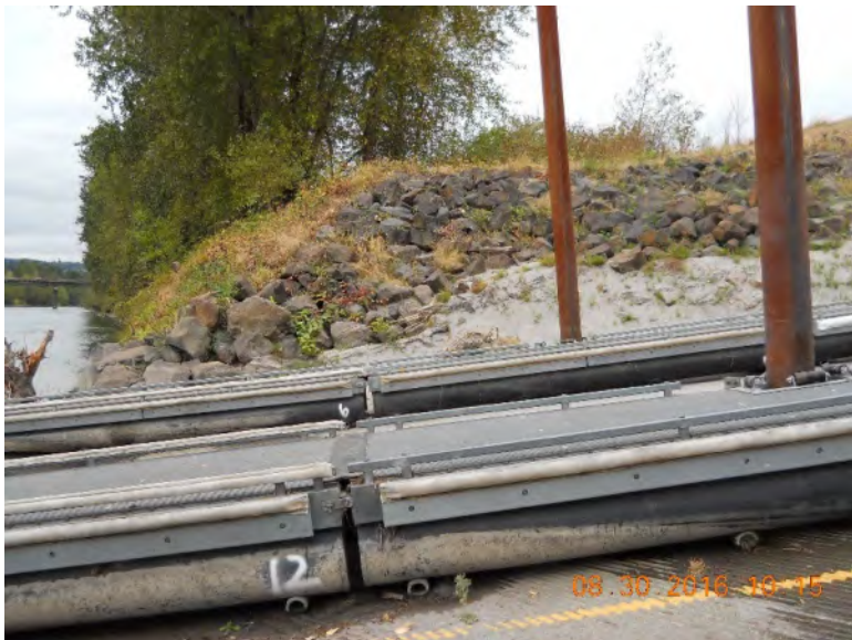
Photo 7 – Boarding floats and marks from sediment deposition
