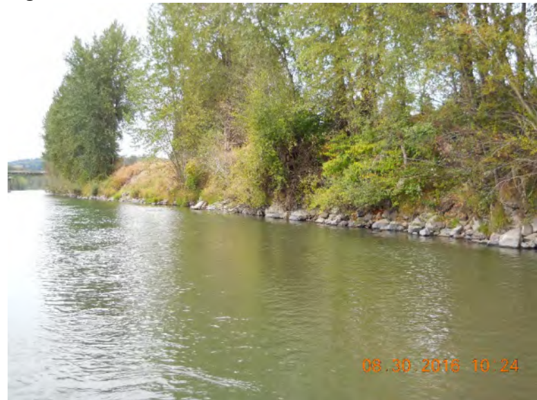
Photo 12 – riprap protection along downstream bank
