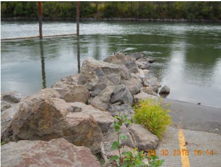
Photo 3 – Riprap protection added after Dec 2015 high water
