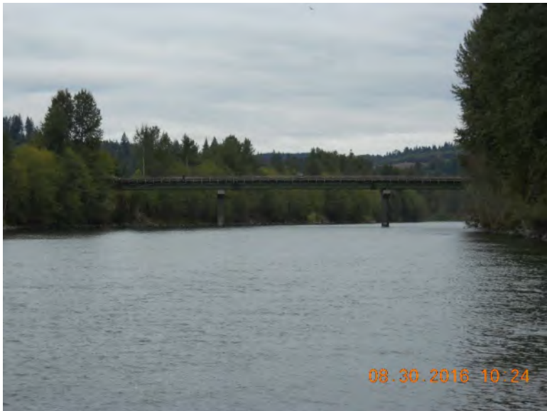
Photo 11 - Looking downstream at Hwy 411 bridge
