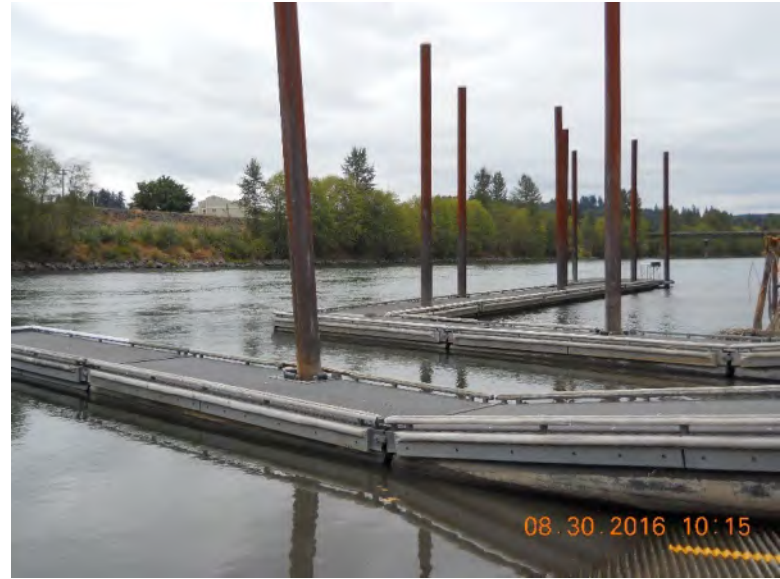
Photo 6 – Boarding floats (foreground) and transverse float (background)
