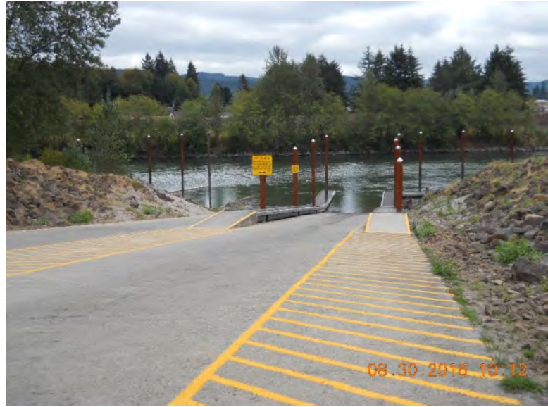
Photo 2 – View from top of ramp
